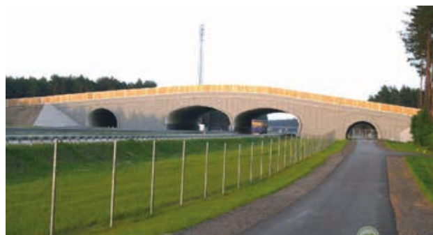
Fig. 25 The best top passages have been built up to now on the A2 motorway, section: Nowy Tomyśl-Świecko 120
