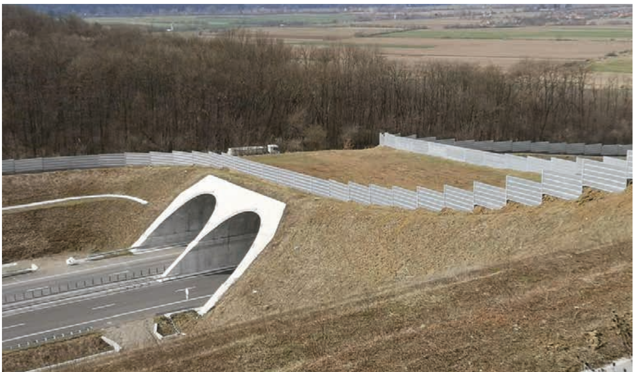
Fig. 26 The first green bridge ever built in Romania - Lugoj-Deva highway, close to Branişca village © Cristian-Remus Papp
