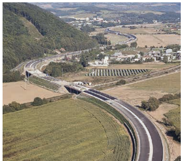
Fig. 42 Dual carriage way R2 from the village Pstruša onward. The road is over many kilometres located on an embankment without any mitigation measures for wildlife. Thus, the important mountain range Poľana on the left of the picture is completely isolated from the south of Slovakia (and Hungary). GPS: 48°32'57.9"N 19°19'32.2"E
