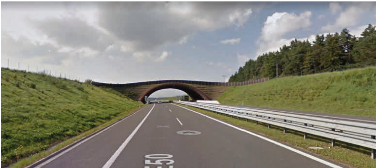
Fig. 27 Green bridge Mengusovce in Slovakia. GPS: 49.043605, 20.391450 © Google maps, 2018
