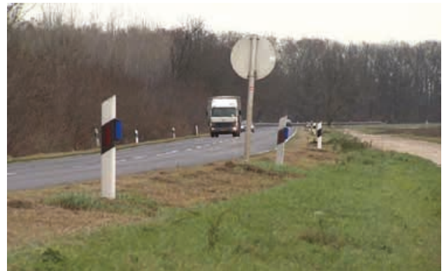
Fig. 22 Blue retro reflectors installed on odometers on Main Road 1 in Hungary, successfully reducing wildlife collisions. Area surrounding GPS: 47°50'59.4"N 17°27'00.1"E
