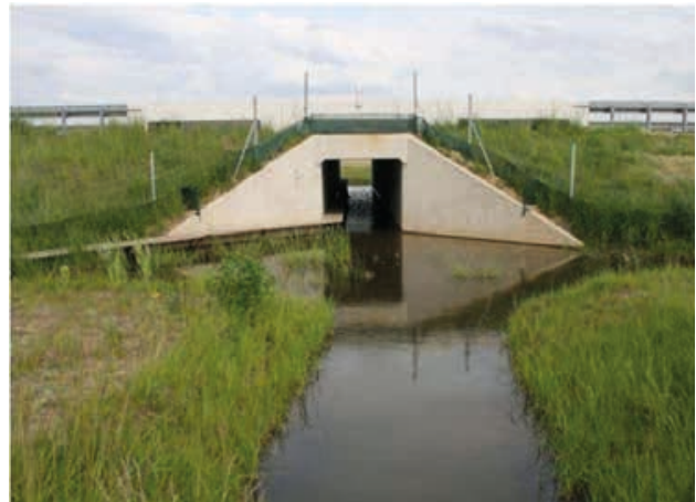
Fig. 38 Underpass for small animals permanently flooded by water 129
