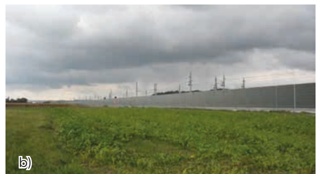
Fig. 44 a) Motorway A1 crossing the wildlife corridor in St. Georgen, OÖ; b) noise protection panels along the high-speed railway in St. Georgen, OÖ 136
